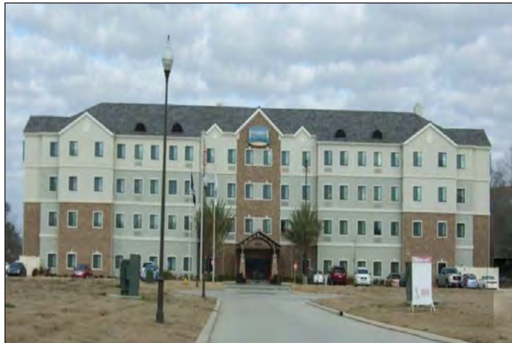
Staybridge Suites Lafayette Airport
