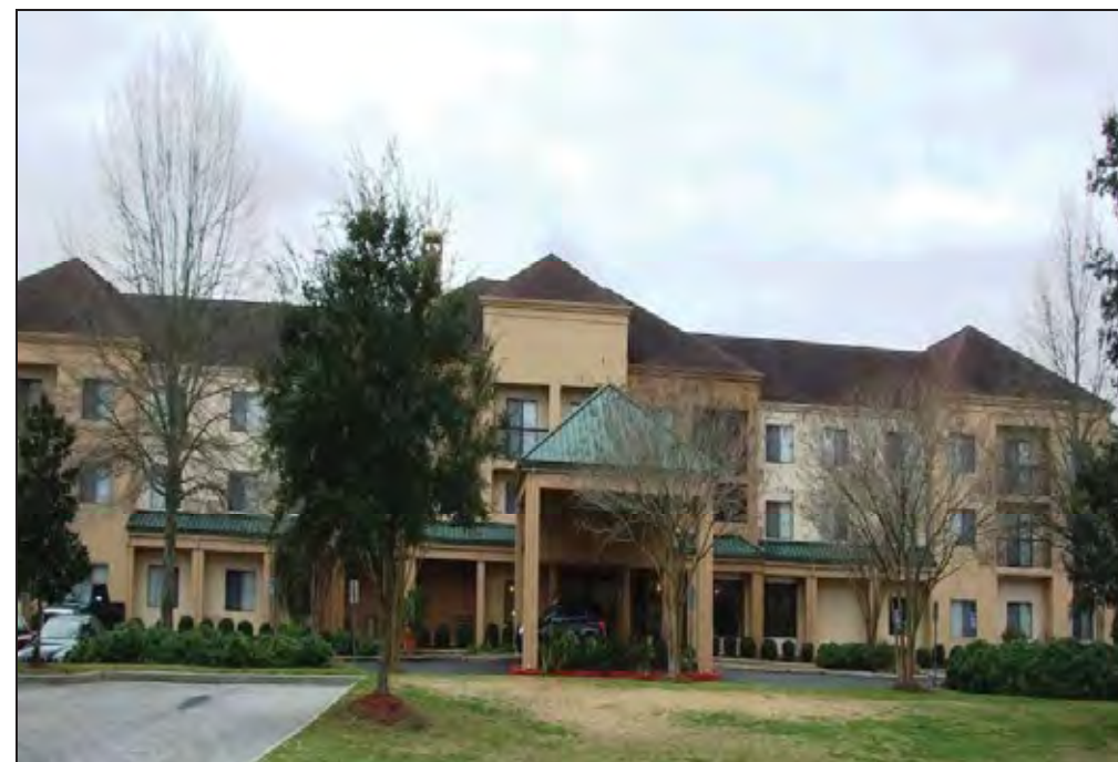
Courtyard Lafayette Airport
